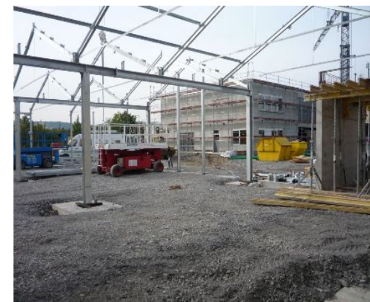
Raiffeisen market, Pforzheim, Germany
